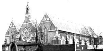
Our Lady of Reparation
